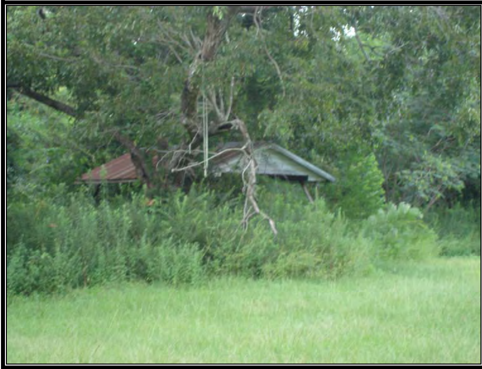
Dilapidated shed on subject property
