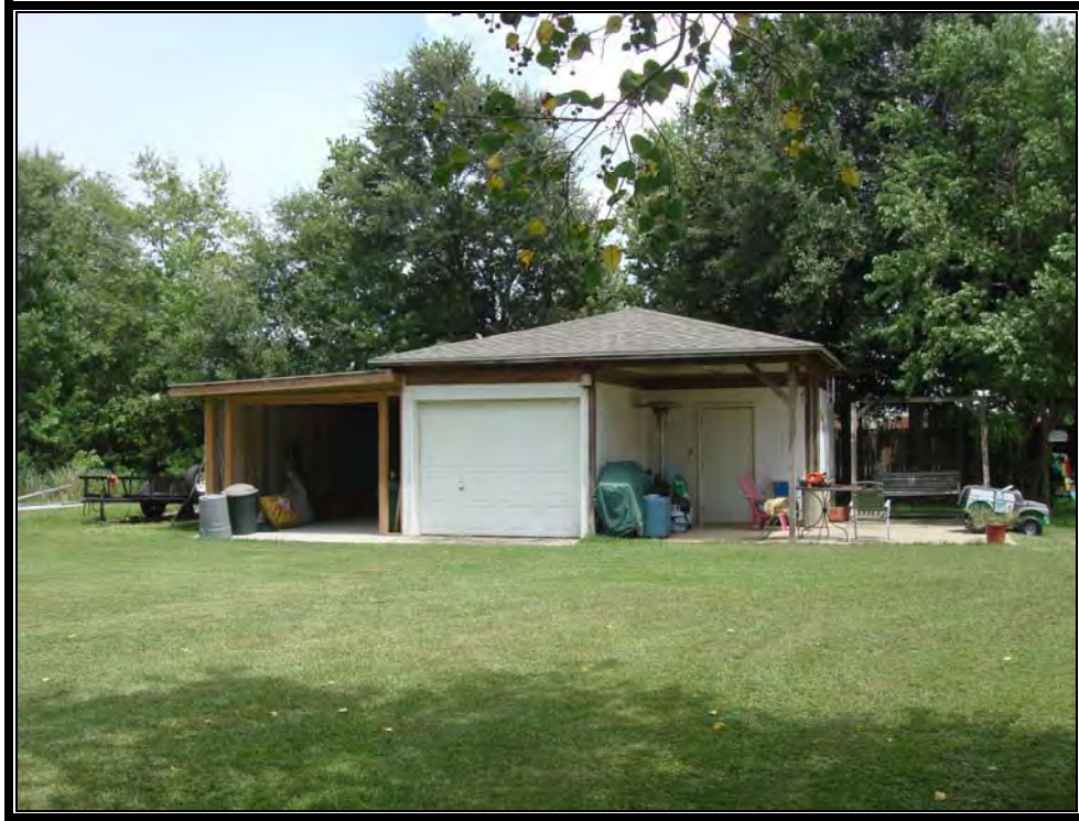
Detached carport and garage, eastern view
